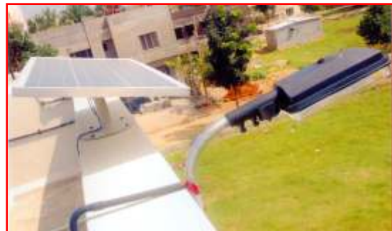
Solar Panel for lighting
