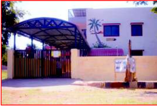
Entrance to Building from road
