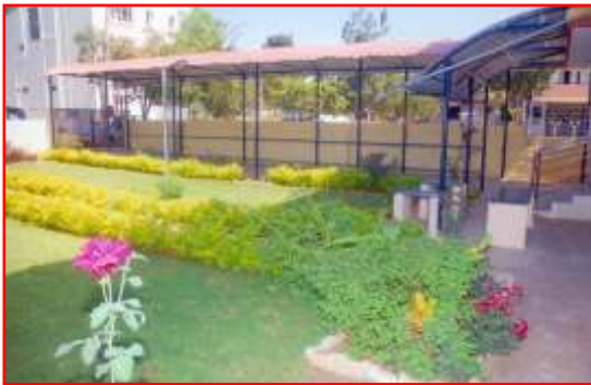
The covered passage leading to the building
